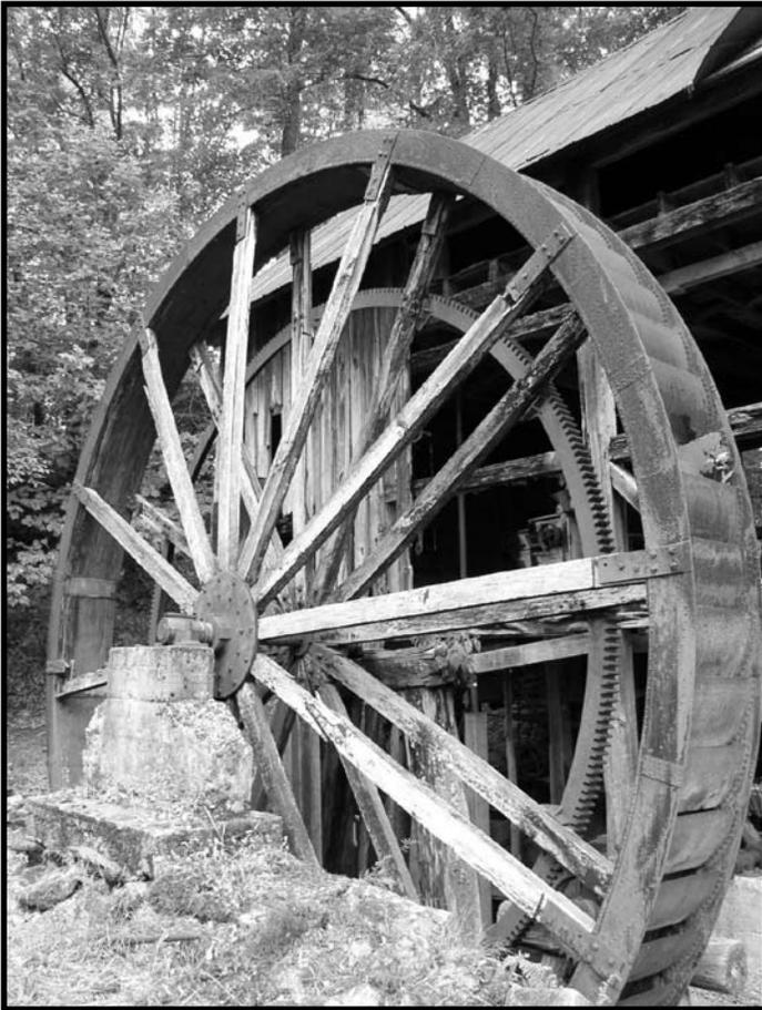
*The condition of the Francis Mill at the start of the July 2004 workshop would have given many people pause. Here you can see the deteriorated state of the water wheel and the poor condition of building's east side. Photo by Mark Slater*
