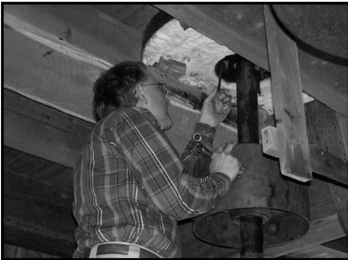
Millwright John Lovett, under the bed stone, inserts the adjustment bolts for the wooden bearings that will keep the millstone drive shaft snug. Photo by: John Lovett.
