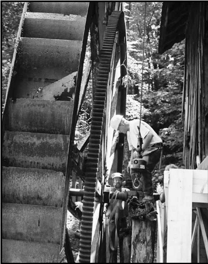
*Lou Mogavero and Will Hines attach the boom crane cable to the wheel before it is lifted from its precarious angle and gently set back down on a new, temporary support. Photo by Jamie Donahoe*
