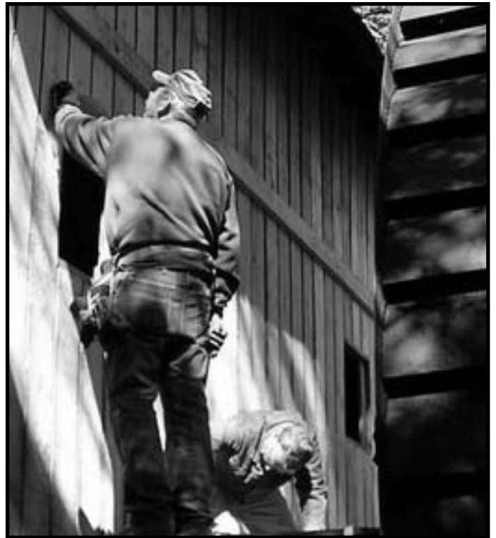
Tim Timbes and Jerry Donahoe install battens on the east side of the mill on a glorious October day in 2006. Photo by Tanna Timbes.
